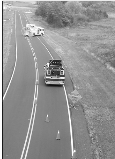
Example of cones and signs as traffic control at a roadway incident.
